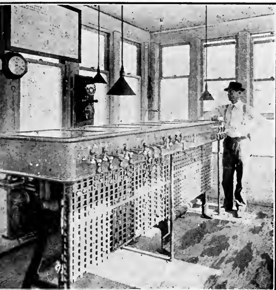
Interior view of Electric Interlocking Tower No. 3 of Key Route
